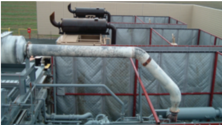
BBC-EXT-R-2" Sound Curtains enclose pumps and compressors.
